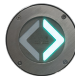
ESCAPE ROUTE TO THE RIGHT
